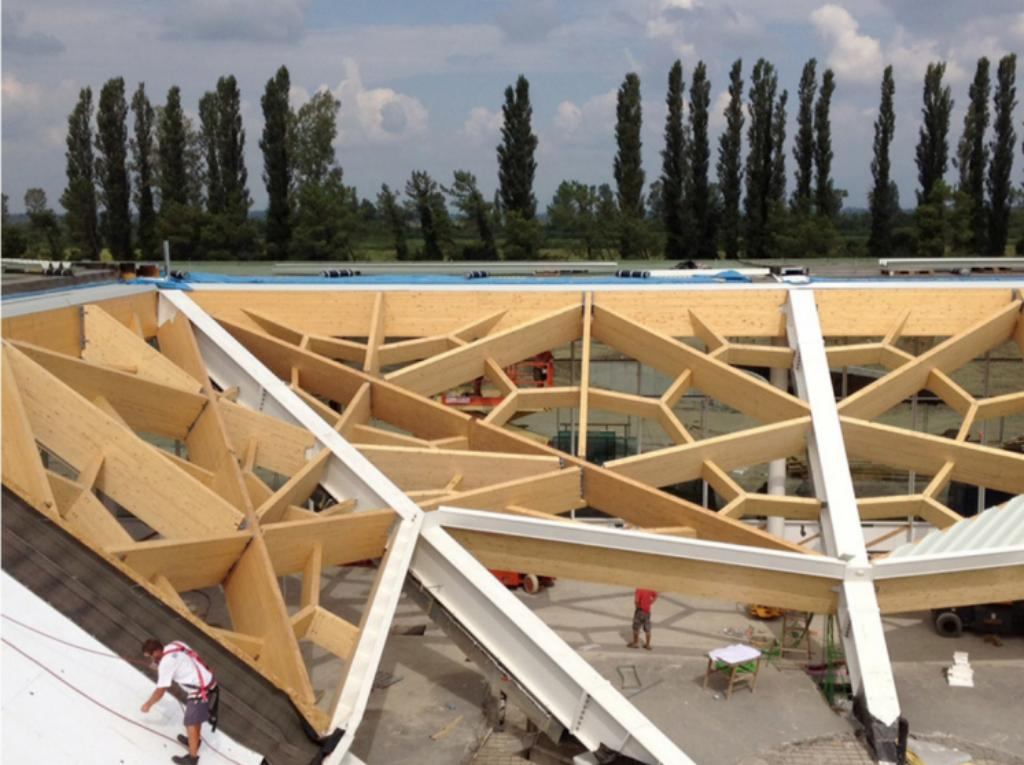
Roof construction for the airport in Kutaisi, Georgian Republic. Gluing of the beams on site with the innovative HESS LIMITLESS System.
