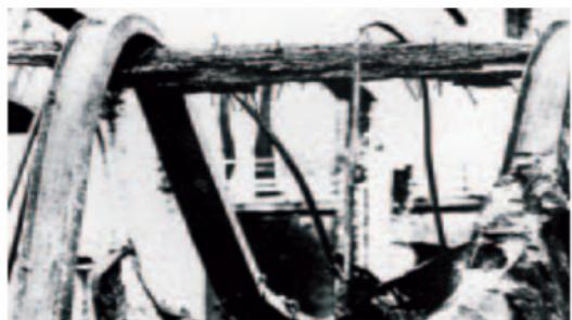
Steel beams have melted and collapsed over charred timber beam which, despite heavy damage, remains in place.
